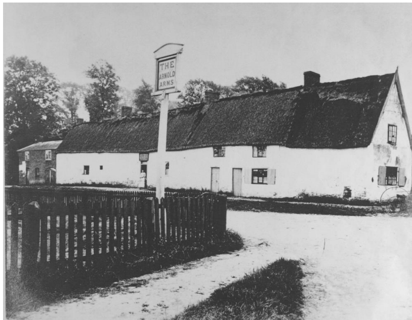
This photograph, taken about 1880-90, shows a cob and thatched building. 19
